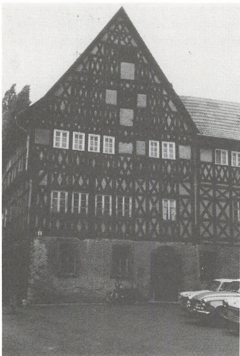
Gammelt hus under restaurering i Arnstadt
